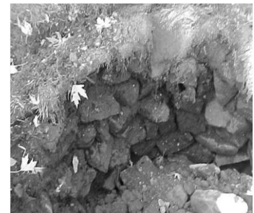
Figure 3. Collapsed Cesspool
